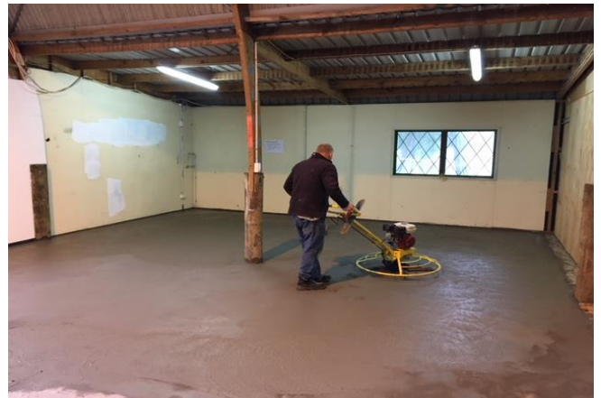
New concrete floor going in
