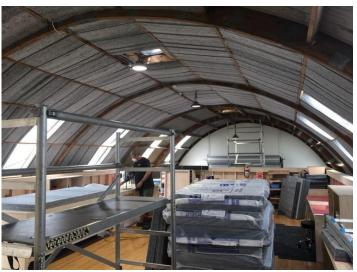
Our shed has been further developed this month, with the installation of Insulation in the metal roof. This will help keep the shed warm in the winter and cool in the summer. It has also improved the acoustics with some of the machinery noise, being absorbed by the insulation material.
